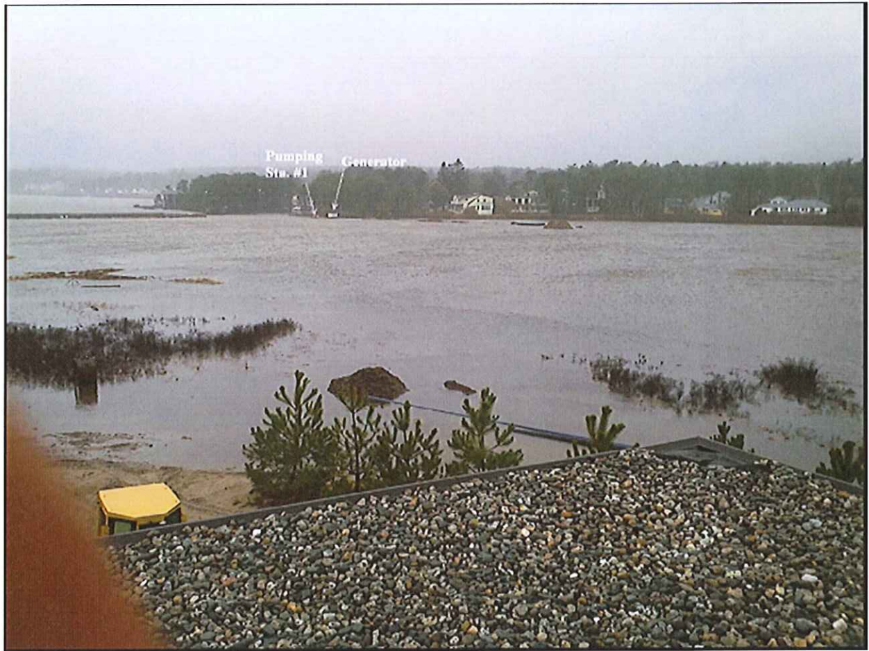
Figure 4-3: Photograph of PS#1 during Present Day Flooding
