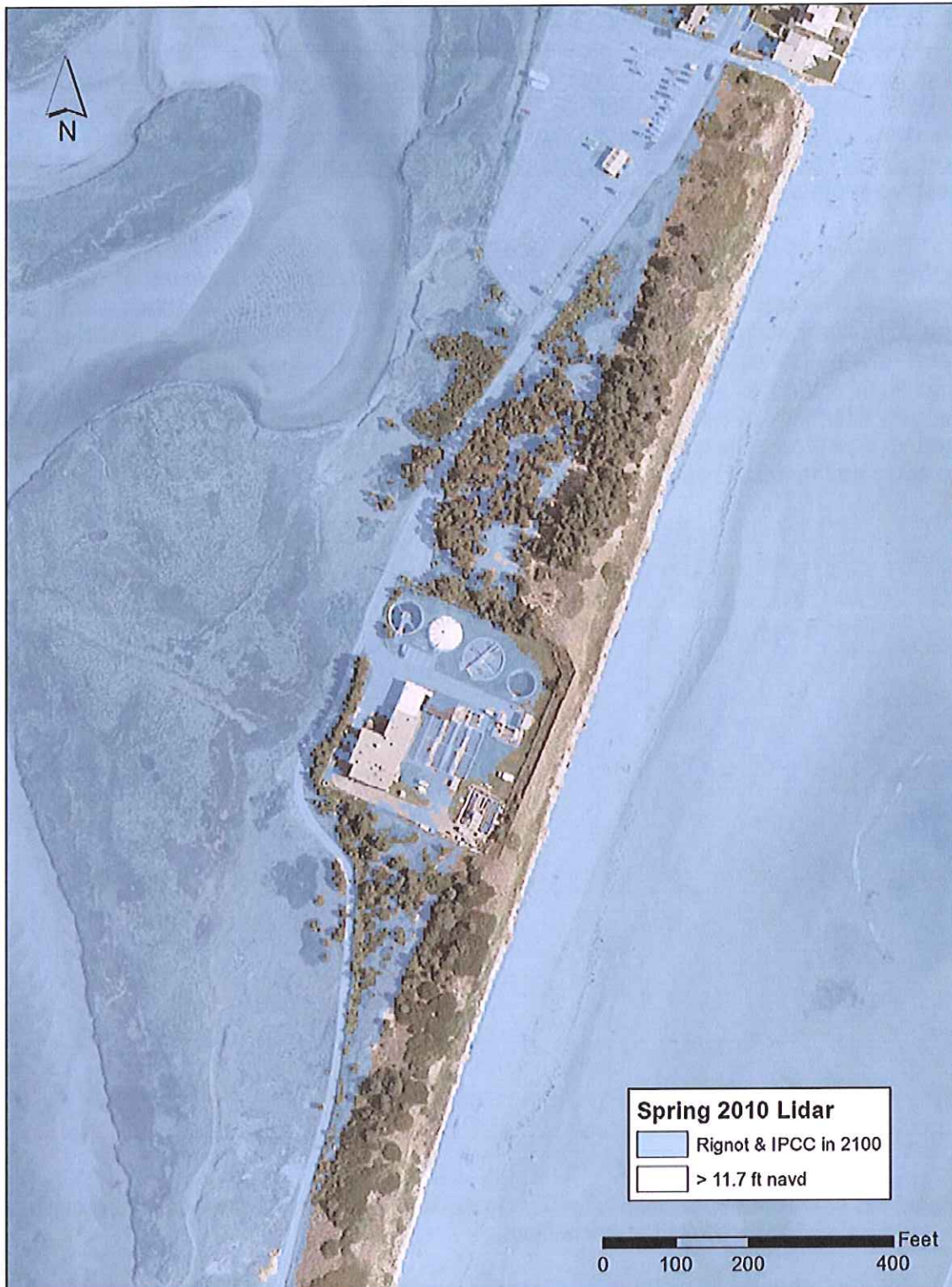
Figure 11. Aerial photograph from 2010 showing the areas that are inundated by flood waters for a 100-year storm event (11.7 feet NAVD) based on IPCC predicted sea-level rise increase in 2100 including updated input for ice sheet contributions (Rignot, et al. , 2011). The areas shaded in blue would be under water during the storm event. Topographic and bathymetric data utilized for this representation were derived from the 2010 LIDAR survey.
