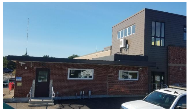
Photo 1 – Control Building North Wall
