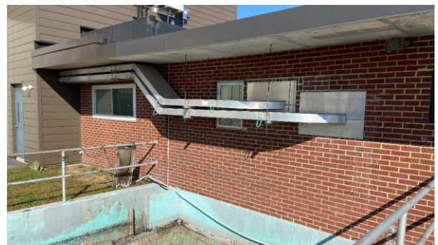
Photo 3 – Control Building South Wall
