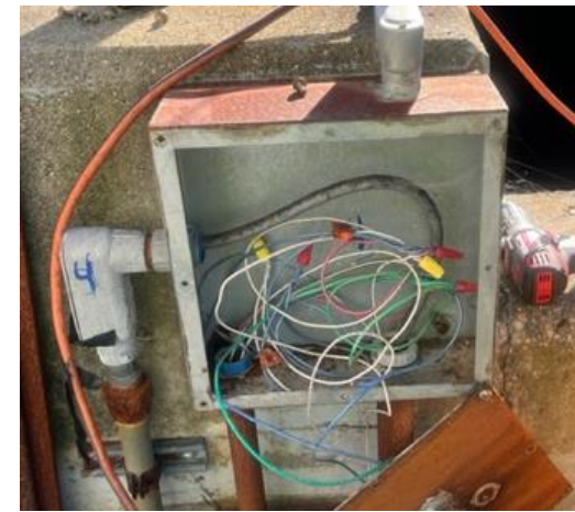
Pull Boxes at Digester No.2 (not shown on dwg)
