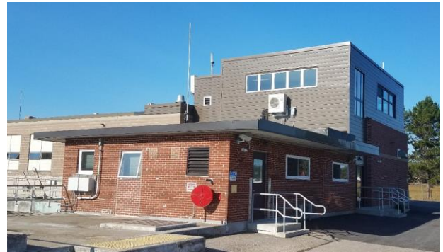
Photo 2 – Control Building East Wall
